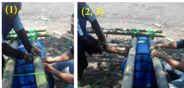
Figure 5. Installation of the Upper Frame Structure
