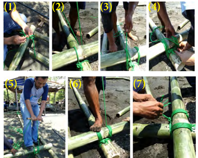
figure 4. Construction of the main structure
